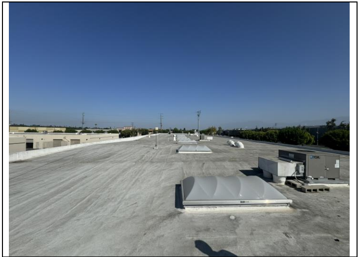
14. View of typical building roof with spray-coated asphalt rolled-roofing.
