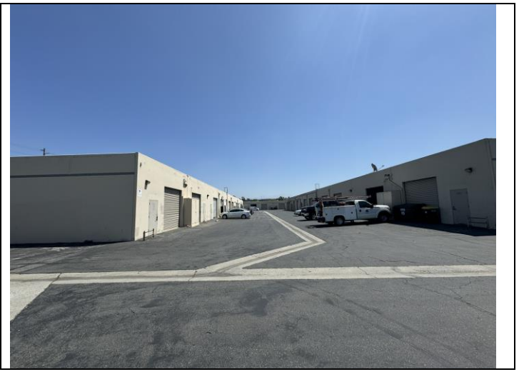
8. View at back of 100 and 120 South 6 th Avenue buildings, looking southeast.
