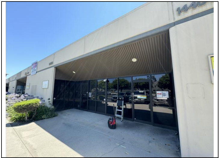
4. View of Property building at 14404 Valley Boulevard, looking west.
