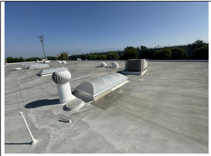
15. View of typical roof vents, penetrations and sun lights with penetration mastic >1% asbestos.
