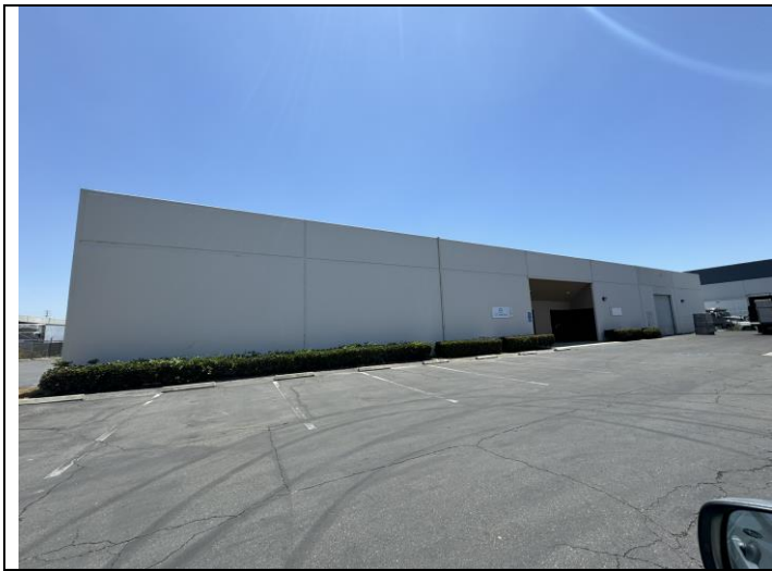
3. View of Property building at 156 South 6 th Avenue, looking southwest.
