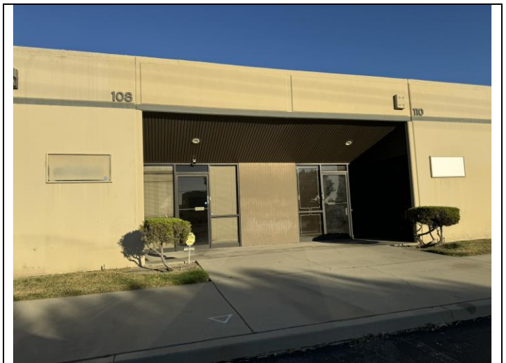
6. View of Property building at 100 South 6 th Avenue, looking southwest.
