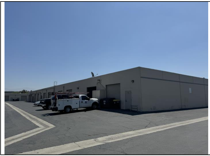
7. View at back of 120 South 6 th Avenue building, looking south.
