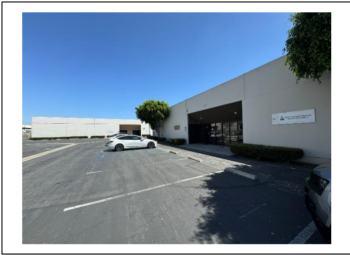
1. View of Property building at 172 South 6 th Avenue, looking west.
