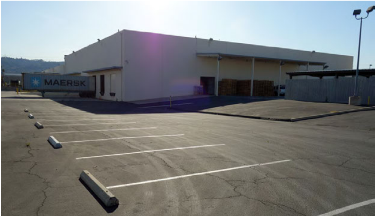
Partial views of south and west building elevations showing building addition area.
