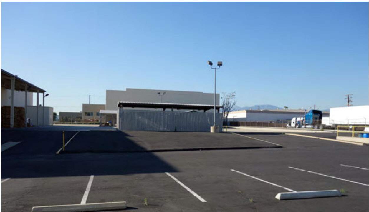
View of structures to be removed to accommodate building addition and new parking areas.
