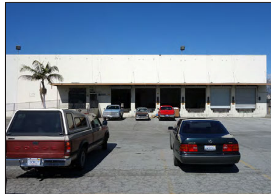
View from southeast of the site looking northwest at part of the commercial building on the subject property.
