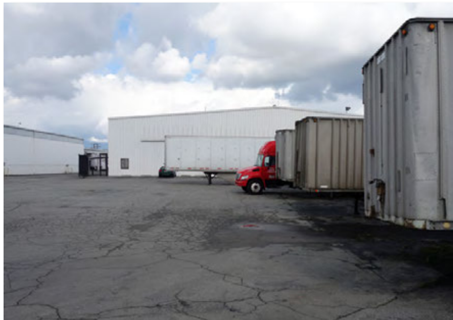
View looking north from the site showing the vacant metal industrial building at 17788 Rowland Street.
