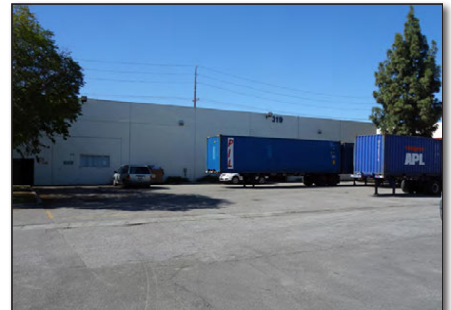
View from southeast of the site looking southwest at the distribution business at 319 Vineland Avenue.
