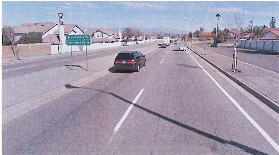
COLIMA RD - LOOKING N/E TOWARD HALLIBURTON RD (SEGMENT WITH SERVICE ROAD ISLAND)
