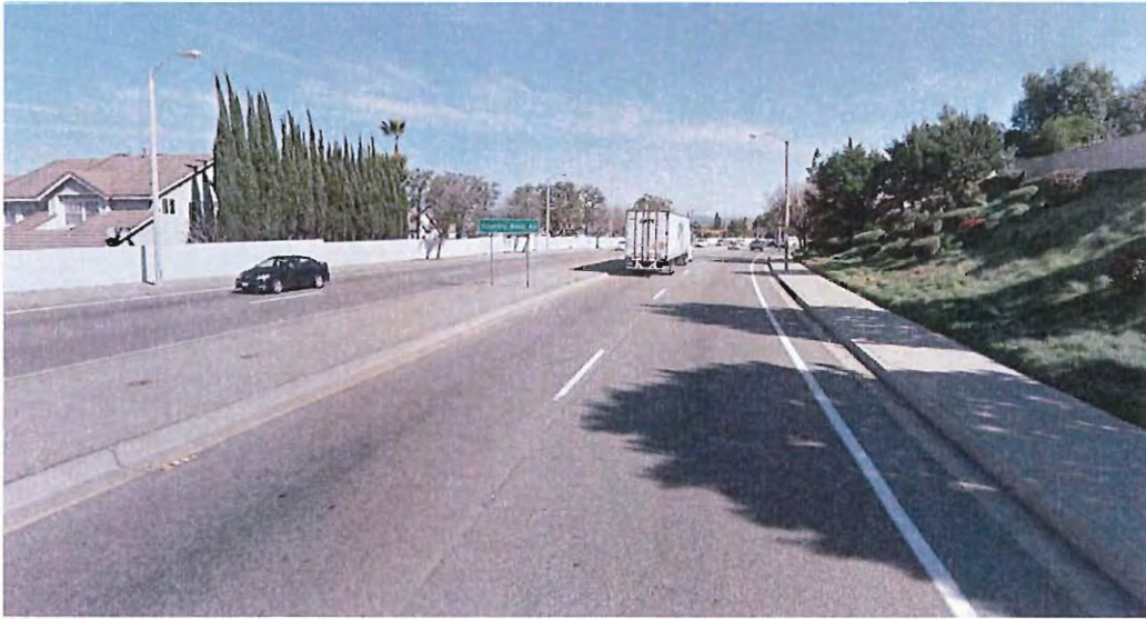
COLIMA RD - LOOKING N/E TOWARD COUNTRY WOOD AVE (SUPER-ELEVATED ROADWAY SEGMENT)
