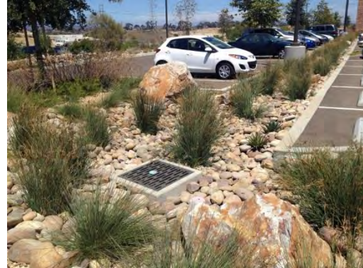
Figure 3-22. Biofiltration in a Parking Lot
