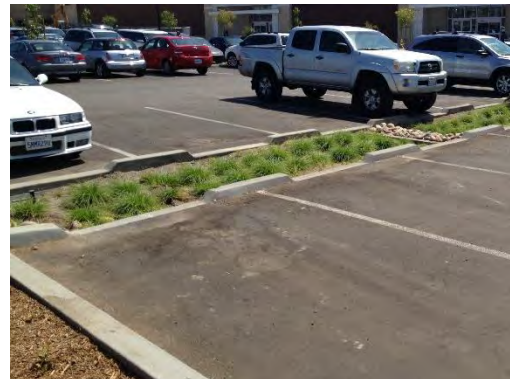
Figure 3-17. Biofiltration in a Redeveloped Shopping Center Parking Lot
