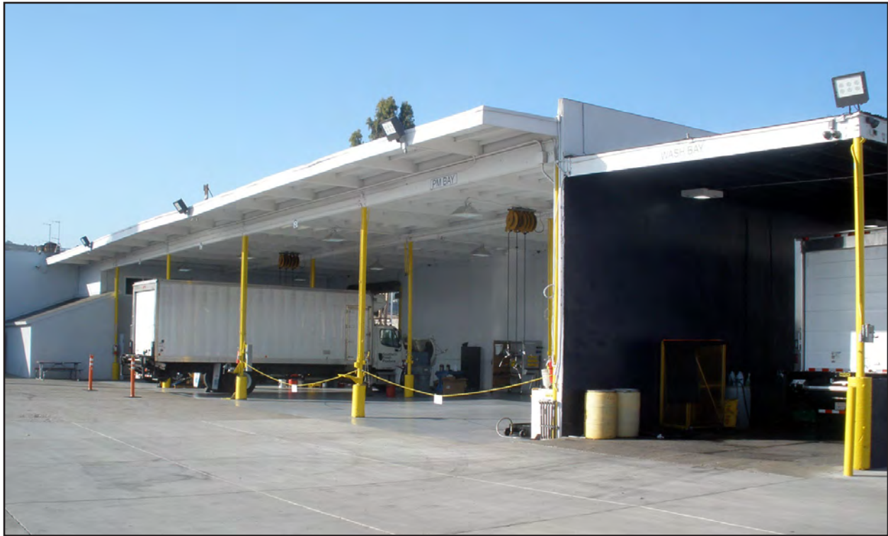
Truck maintenance and wash bays extend from the office building just southeast from the proposed AST location. One of the two AST emergency shutoff switches will be located near the post at the far right of the photograph.
