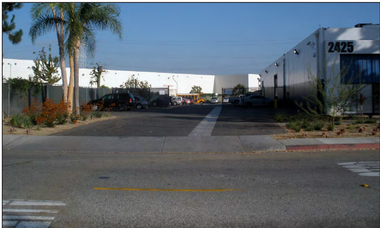
Entranceway and parking lot on the southeast side of the industrial building, viewed across Kella Avenue.
