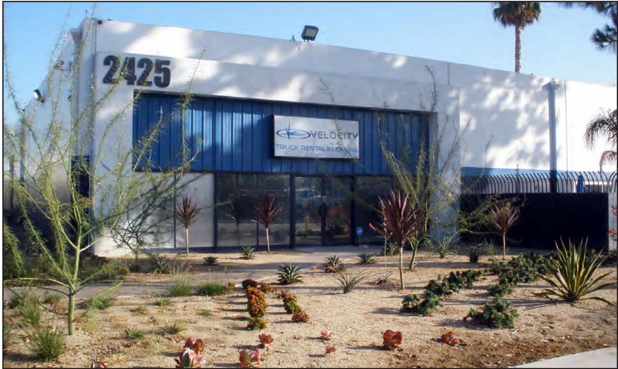
Front of existing industrial office building at the project site, viewed toward the north from Kella Avenue.
