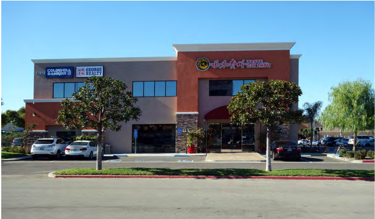
View looking west of the east exterior of the building containing the project site; the entrance to the unit is at the bottom right of the building.
