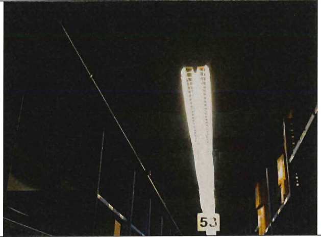
Warehouse Linear Fluorescent T8 Fixture
